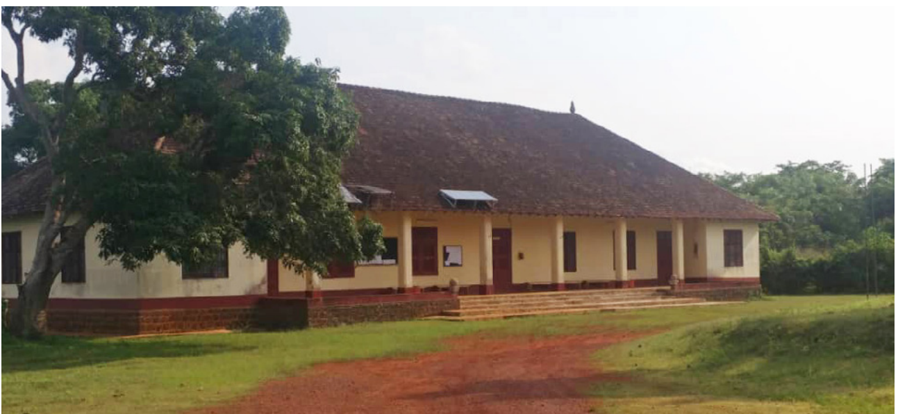
Figure 4 – Hospital building in Doumé
